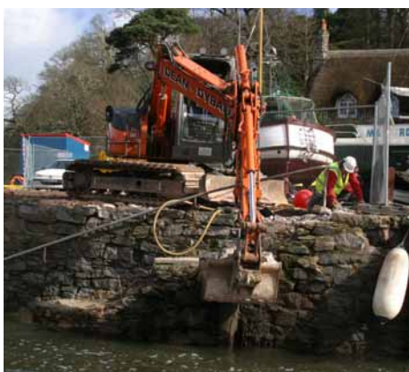
Greenway Quay under restoration
