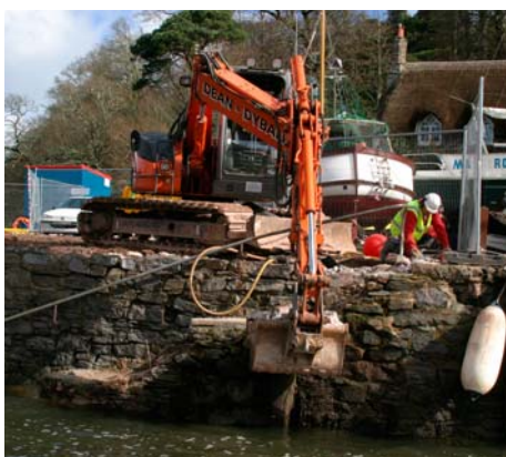
Greenway Quay under restoration
