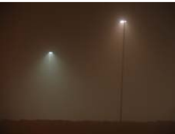
Well directed full cut-off lighting in use at Dartmouth Leisure Centre car park
